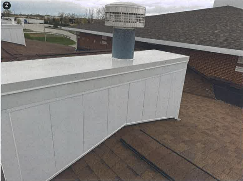
2 New sealant around penetrations on Chimney areas.
