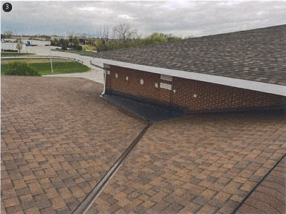
3 EPDM Cricket areas removed and new EPDM installed
