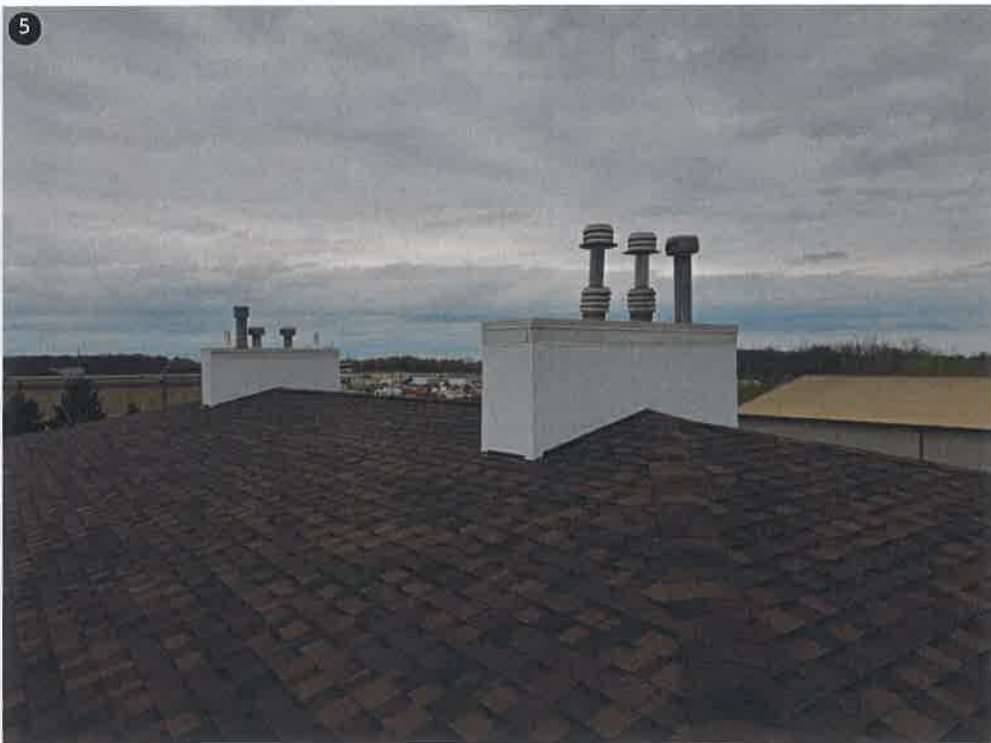
Upper Roof Metal Cladding installed around Chimneys
