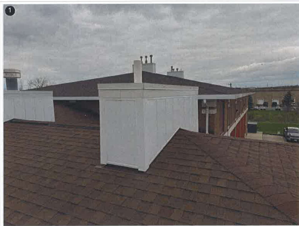
Complete Installation of Chimney Metal Cladding
